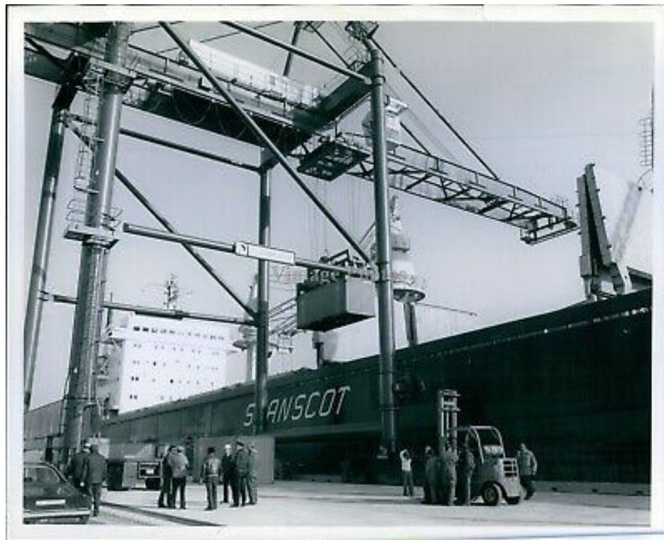
Photo V-2: Duluth Container Quay Crane (Ron Johnson)
