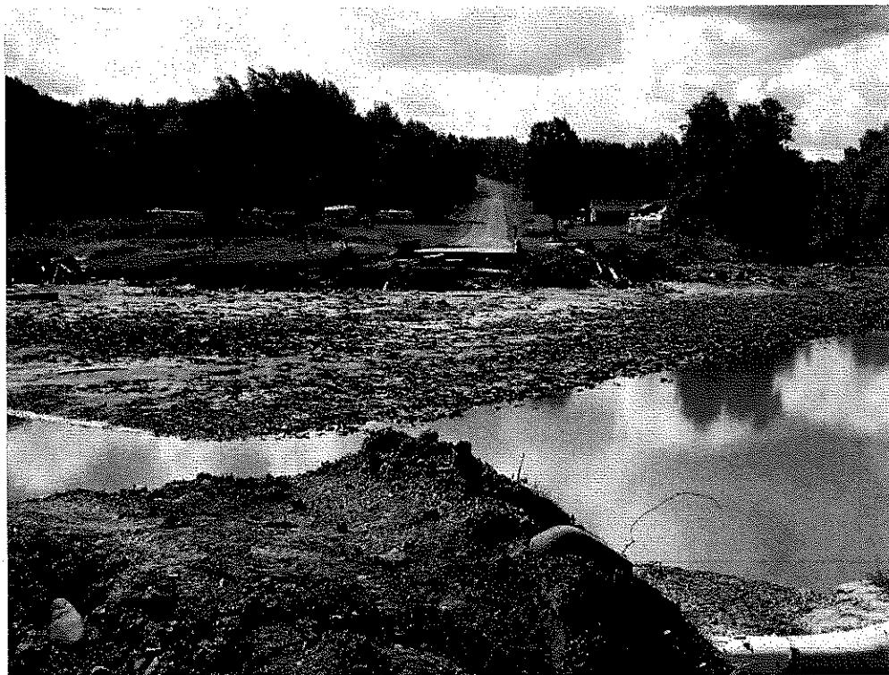
After storm where County Hwy A bridge was washed away.
