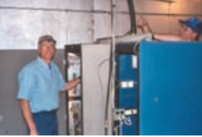
Engineers dismantle old equipment at WLSU-FM/La Crosse.
