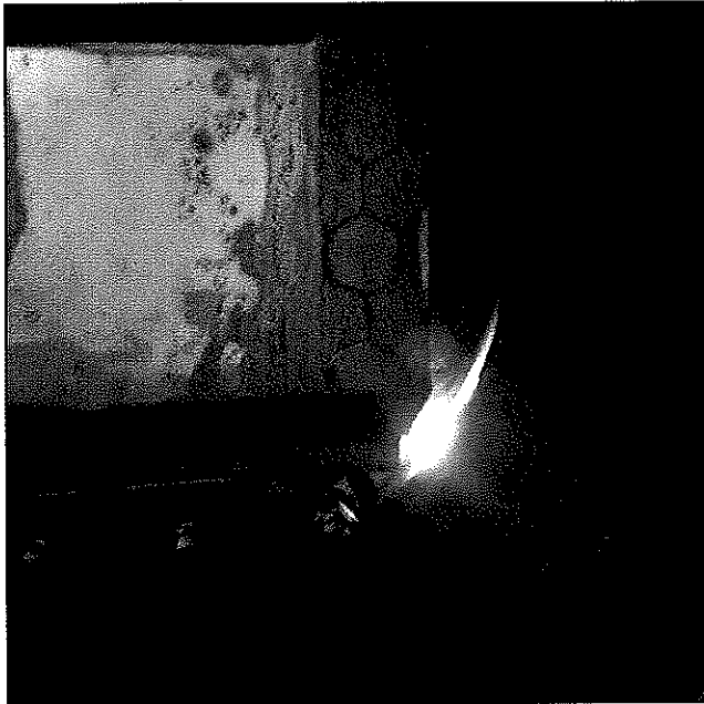
Figure 23: Light shining through the gap between the spent slide valve gate and seat ring.
